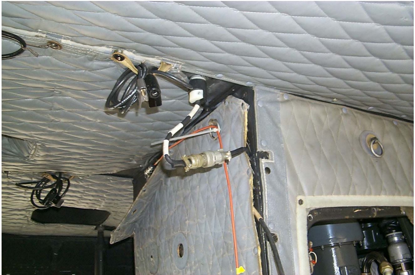
Figure 2. DC Power Cable Installation
