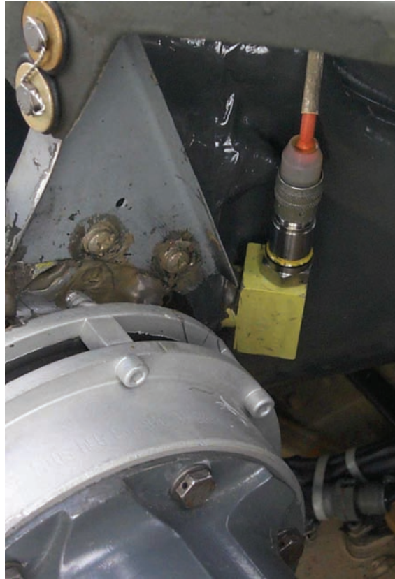
Figure 18. No. 1 Input Module Accelerometer Installation (ACC1)
